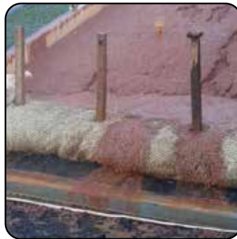
Fig. 6: 20" Straw Wattle (70% Removal Efficiency)
