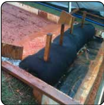
Fig. 2: 12" SiltSoxx™ (97% Removal Efficiency)
