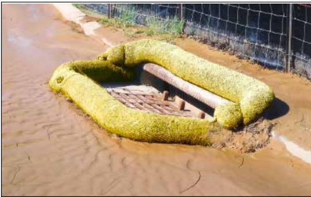
Filtrex® SiltSoxx™ for Inlet Protection
