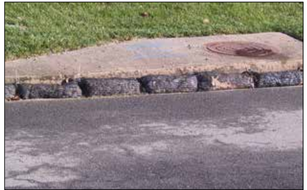
Typical rock bag installation for inlet protection
