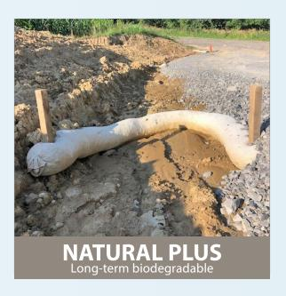
Filtrexx SiltSoxx® is the quickest, easiest and most cost effective solution for sediment control.
